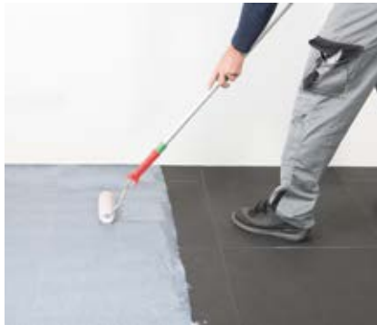
Application of the pressure sensitive adhesive
