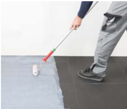
Application of the pressure sensitive adhesive
