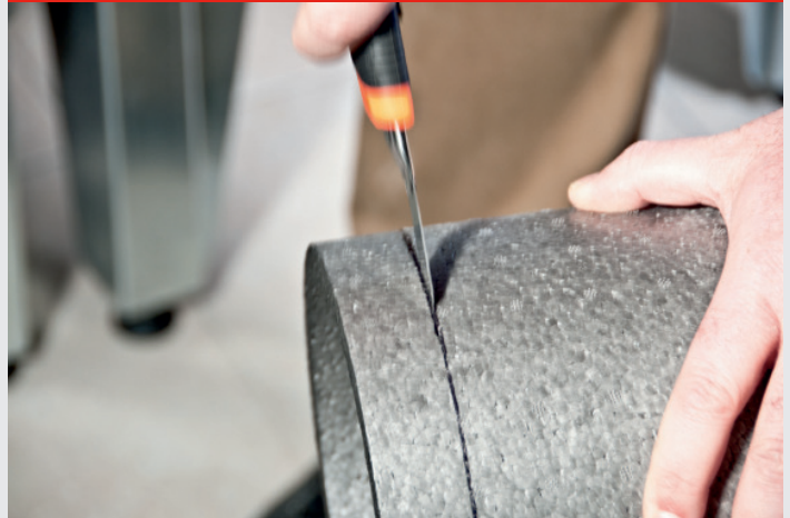
Cutting ComfoPipe to Length
