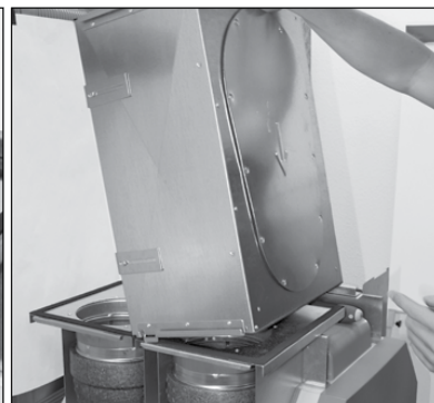
9. Place ComfoWell on the end plate
