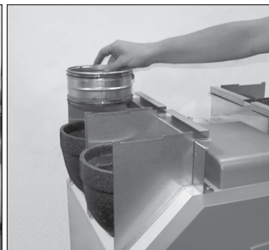
6. Insert the 160 mm nipple into the CA 350
